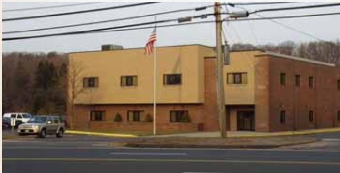
Visible mechanical equipment
