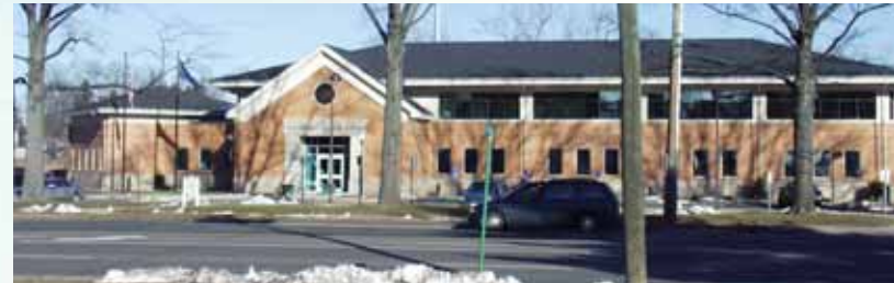
Town Center - Municipal Building
